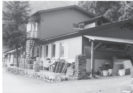
Picture18. Factory of co-operation in Asyuu settlement.
